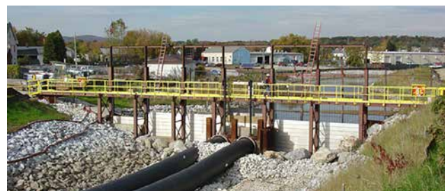
Dredging the East Branch in Massachusetts
