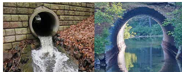
Left, poor culvert. Right, good culvert.
