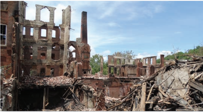
267 Canal Street Building Demolition
