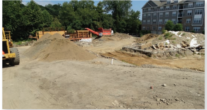
223 Canal Street Environmental Site Remediation
