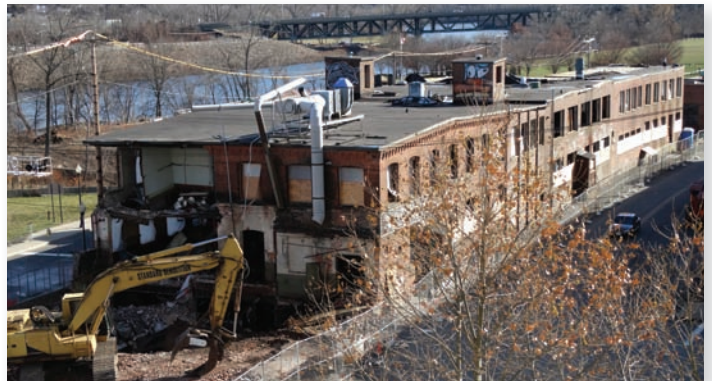
113 Canal Street Chromium Process Demolition
