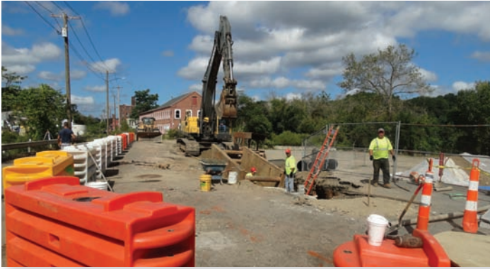
Canal Street Reconstruction
