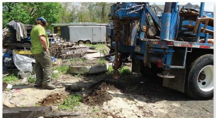
235 Canal Street Environmental Site Assessment
