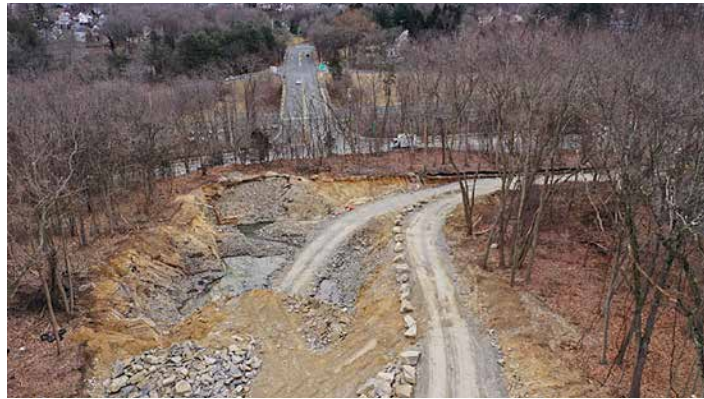
Constitution Boulevard Construction Looking South Toward Rt. 8
