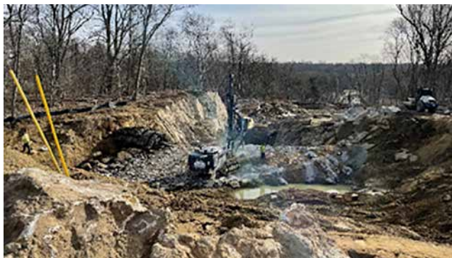
Blasting and Excavation of Rock Materials
