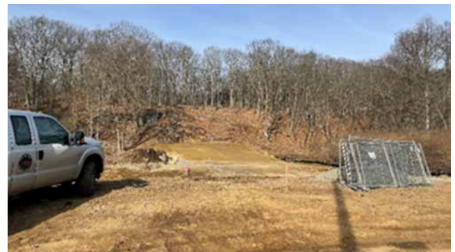
Road Extension North Toward Rt. 108
